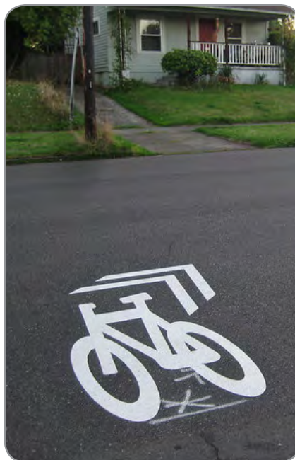
Raleigh has been installing shared lane markings since 2010. Sharrow arrows like this one can also be used to inform bicyclists of an upcoming turn.
